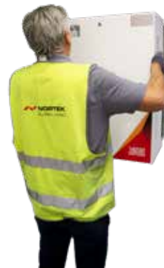
Fig 2h - Sliding front panel on to unit
