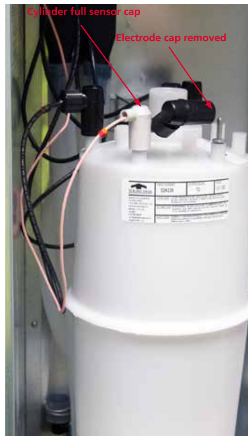
Fig 15 - steam cylinder showing electrode caps
